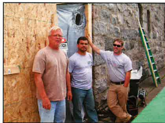
Pictured from left to right: Paul Johnson of Intermountain Technical Services, Mayville, ND; Miguel Garcia and Nathan Wretling of J&N Enterprises, Grand Forks, ND. This photo was taken during interior abatement and salvage of interior bank items.
